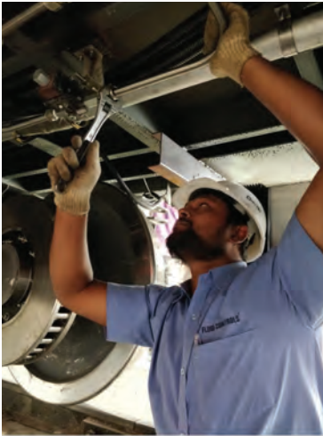
Fluid Controls® Installation Team on Site
